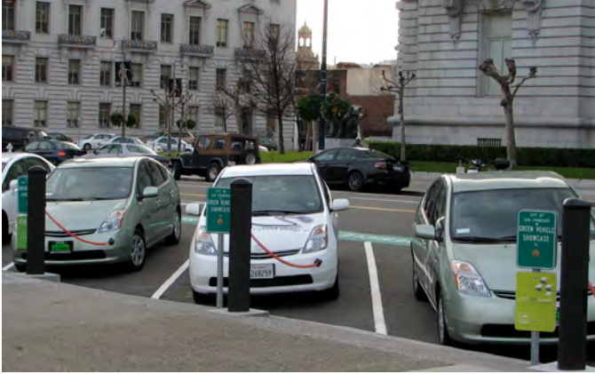
Figure 10. Head-in angled parking spots are good locations for EV charging infrastructure, as with these stations installed in front of San Francisco's City Hall as part of the city's Green Vehicle Showcase in 2009 (Felixkramer/Flickr (CC BY-SA 2.0))
