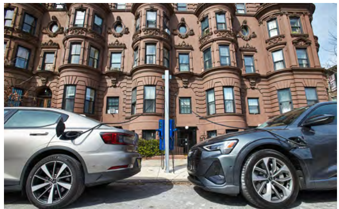
Figure 1. On-street publicly accessible EV charging infrastructure expands access to those who don't have access to private charging facilities in garages or off-street parking spaces (FLO)
