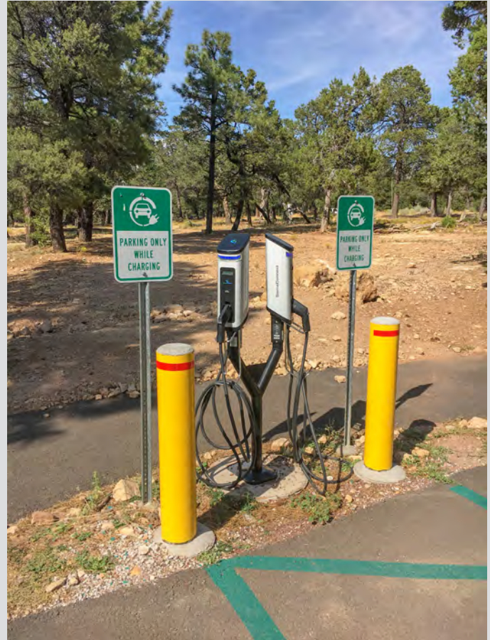
Figure 3. Level 2 chargers at Grand Canyon National Park (Grand Canyon National Park/Flickr (CC BY 2.0))
